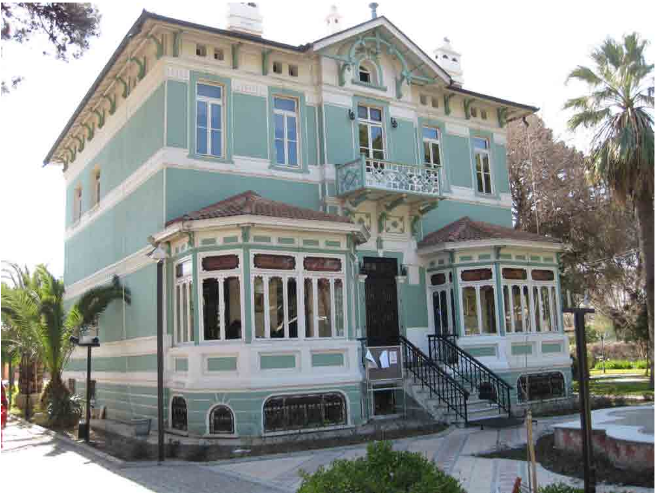
Ege University's Yeşil Köşk (Green House), İzmir (Photograph by Meldan Tanrısal)
